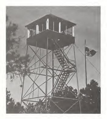
Figure 136. Turkey Butte lookout, an Aermotor MC-24 erected by the CCC in 1937.
